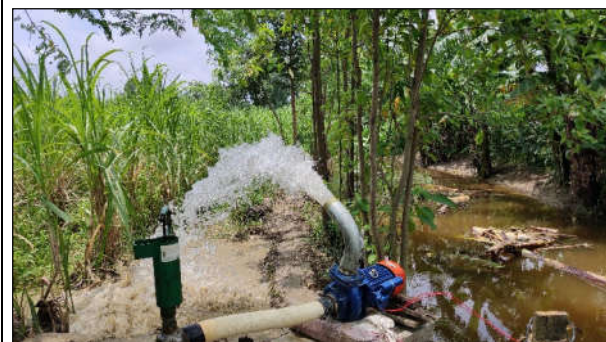
Shallow Tube Irrigation Schemes Installation at Karjanha, Siraha
