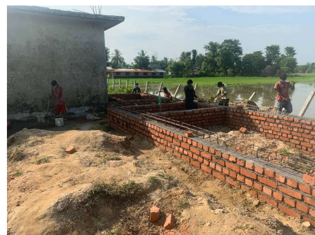
Under Construction of Girls Toilet of Chandra Kamal School, Sunsari
