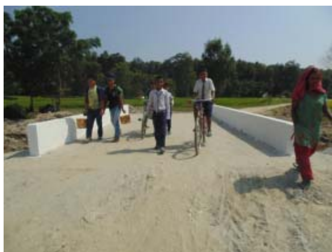
School children passing through culvert which was constructed under 4CA project
